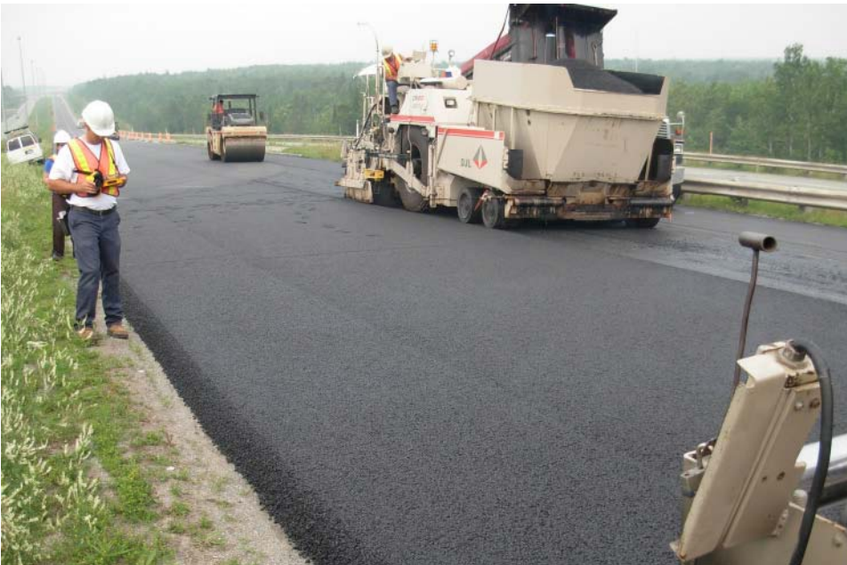
Taking asphalt temperatures during application.
